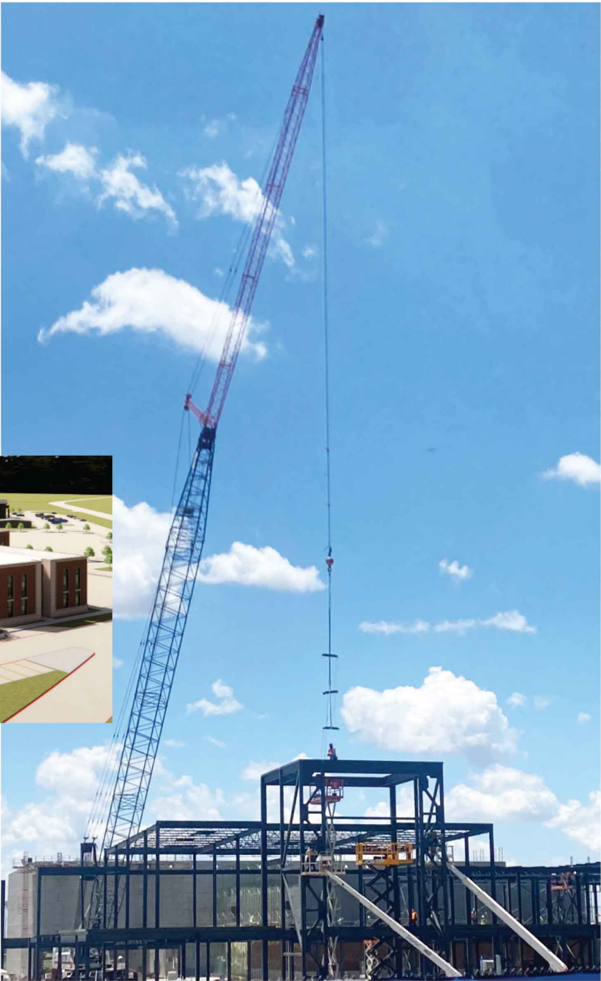
RIGHT: A large crane sets metal beams in place on the tower of the new Sanger High School, as workers weld them in place earlier this week. ABOVE: A rendering of the new high school at completion. LEFT: The secured outdoor courtyard that can be used by students.
