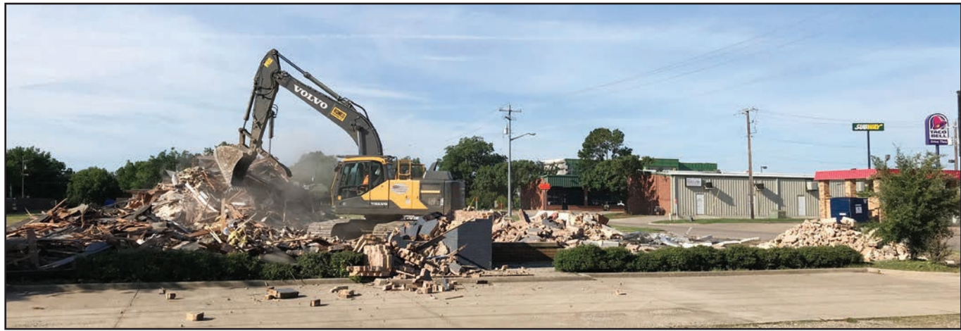
On Wednesday morning a trackhoe separates parts of the demolished building.
