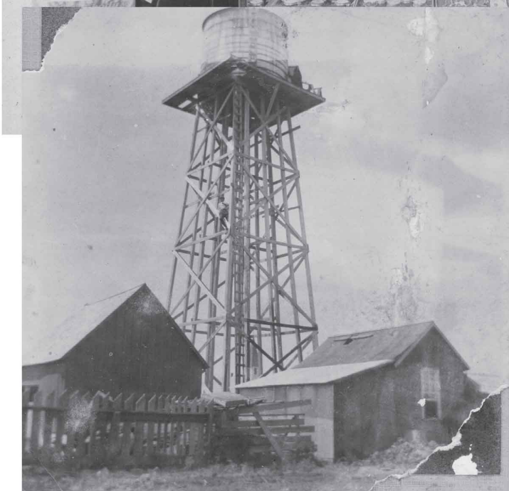
LEFT - Answer Part 2: This is the first public water tower in Sanger that was owned by Dan Davis. The tower was built in 1906 by Frank Thatcher and Charlie Henderson. Henderson was a co-owner with Dan Davis. The wooden tower fell in 1910 and was replaced with a 900-gallon wooden and steel tank on Fourth Street.
