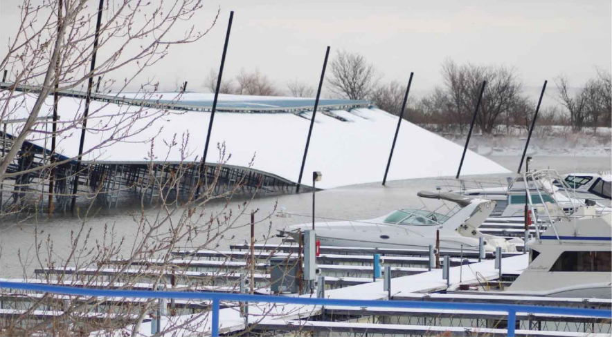
Lake Ray Roberts boat house three collapsed from the weight of the sleet/snow. This was a brand new boat house that was being constructed. There were no boats in the slips and it was replacing the boat house that was completely destroyed in a tornado in May of 2024. Boat house nine sustained damage, as well from the sleet and part of the roof collapsed and some boats were damaged.
