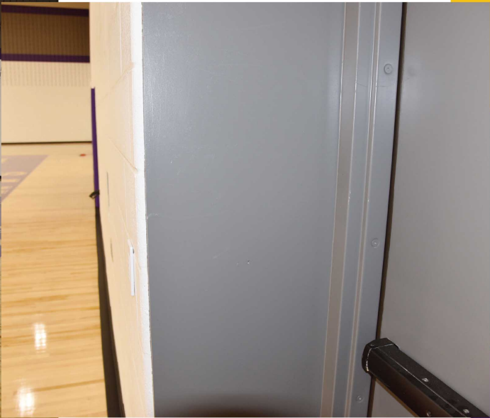
The secondary gym has 15" thick concrete walls/ceiling and is the designated tornado shelter at the high school. It is a new state mandate to have this in all new construction of schools in Texas.
